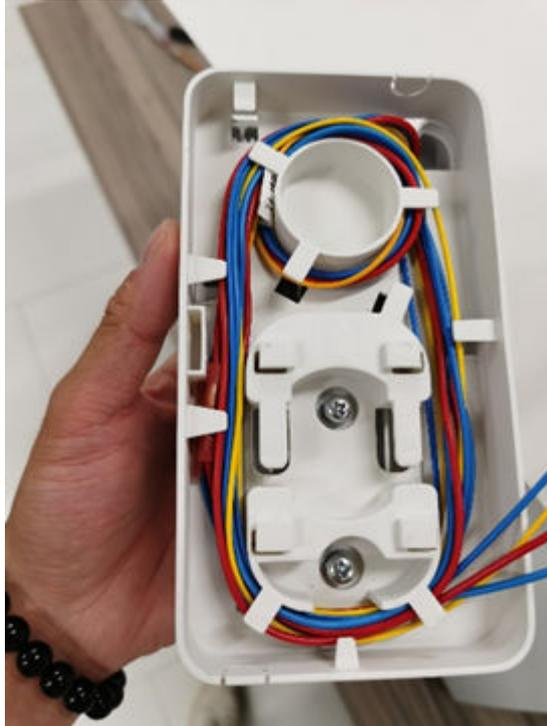
Junction box mounting scenario: If the remaining length of the cable is not enough for a large circle, coil the cable in a small circle and fasten the fiber to the cable tie in the middle of the fiber management tray.
